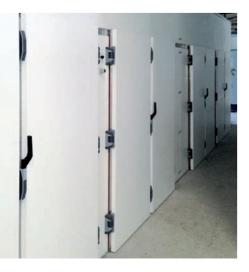
Sturdy and long-lasting: the innovation involves using closed cell fiberglass panels, i.e. seamless, without gaps between the insulating material and the outer coating panels.
